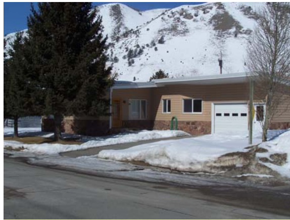
Karns Avenue, single family home
