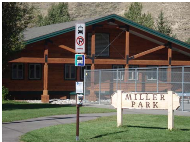
Community Services, Facilities, and Infrastructure are important to community health, safety, and wellbeing.
